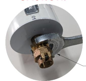
FIRMLY HOLD THE SERVICE FITTINGS WITH A 1-3/8" WRENCH WHEN MAKING THE SERVICE CONNECTION. DO NOT ALLOW THE FITTING AND/OR BARREL TO TURN OR TWIST
